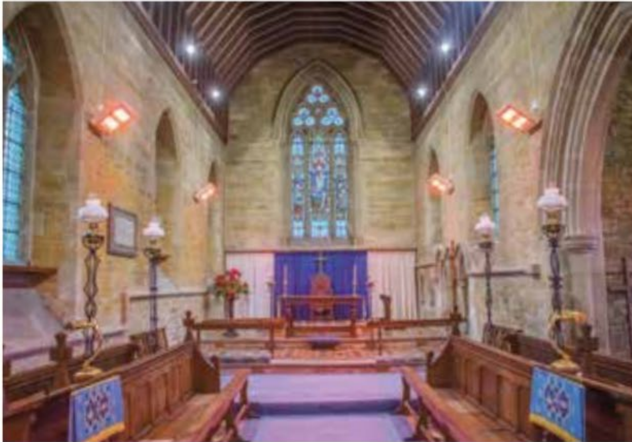
HN Halogen Heaters heating a church in Market Harborough
